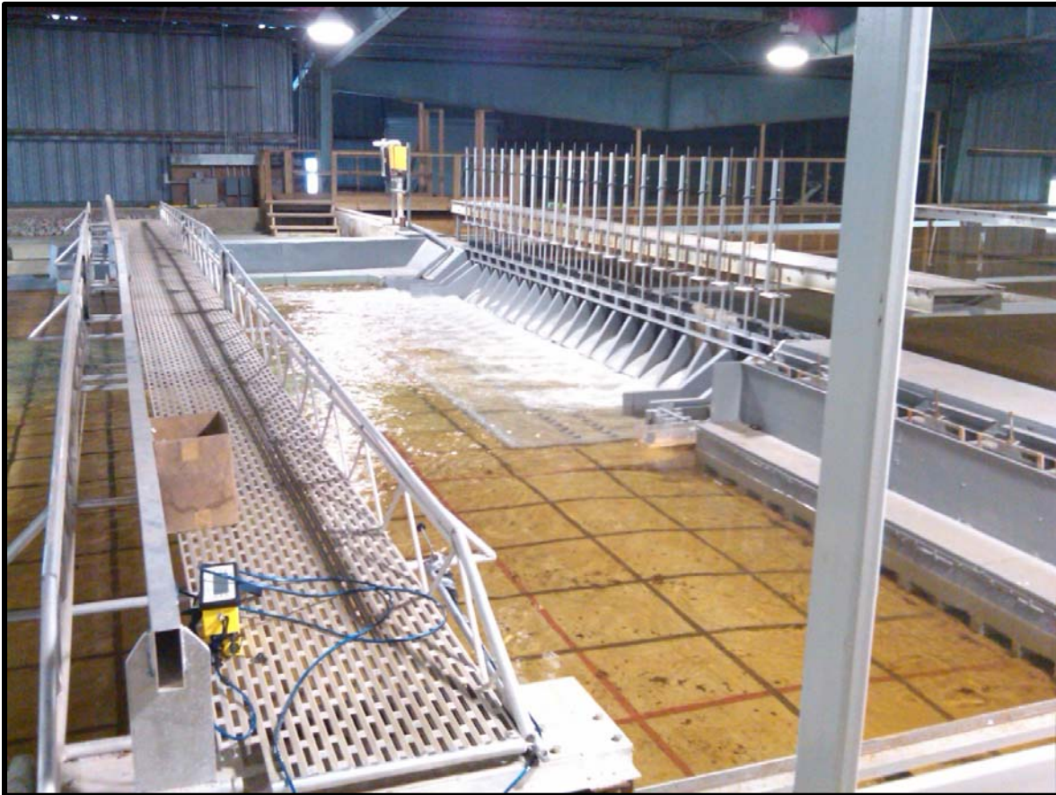
Figure 23. McNary General ERDC Model During Testing in March 2012
