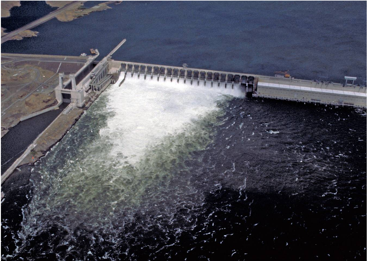
John Day Lock and Dam located on the Columbia River near Rufus, Oregon.
